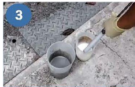
3 Mixing PowerJet powder with the resin inside the hand pump injector.
