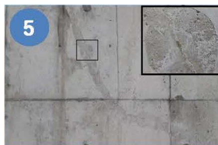
2 Seal the cracks on surface using quick-set epoxy or hydrated cement.
