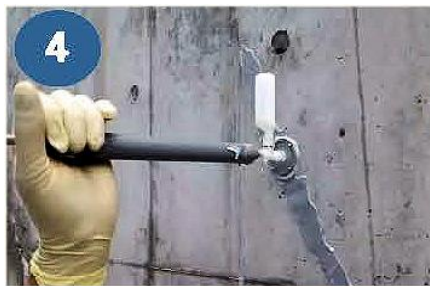
4 Inject PowerJet into the crack
