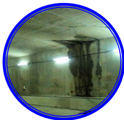
Water Leakage
