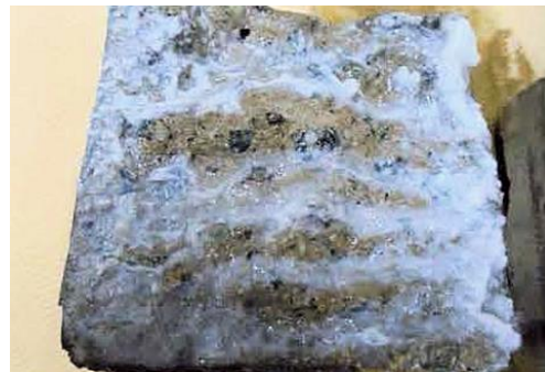
Inside the crack face
