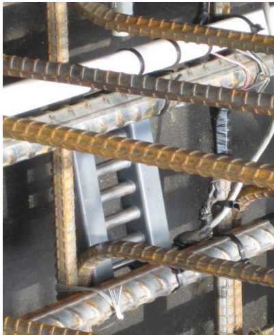
Installation on Wall
