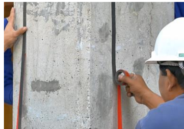
2. Attachment of Betel Guard MMO Titanium Tape
