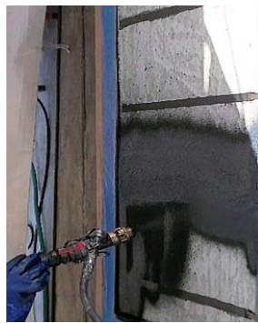
4. Applying Concoat to finish the CP anode system. (right: hand trauanting, right: spray)
