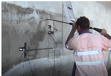
1. Surface preparation by high pressure water
