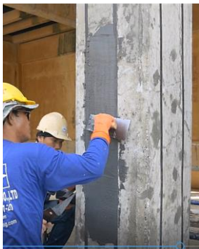
4. Applying Concoat to finish the CP anode system. (right: hand trauanting, right: spray)
