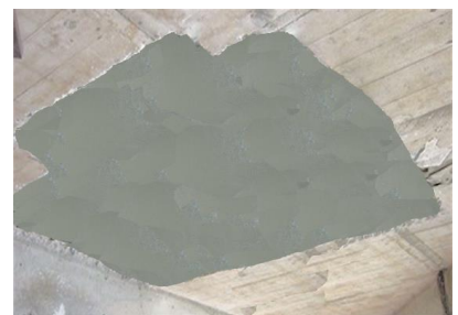
3. Patch with Repair Mortar.
