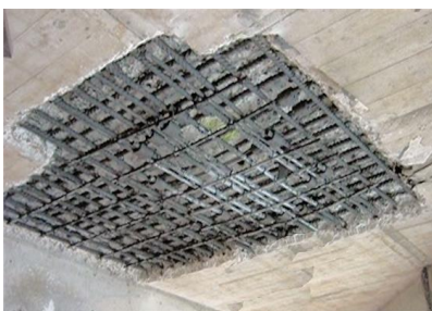
1. Remove damaged concrete
