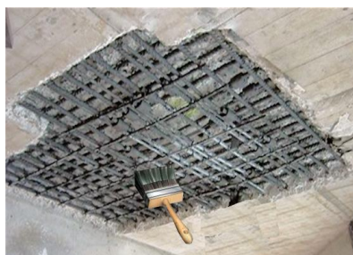
2. Apply Cementex Inhibitor Paste by brush or spray.
