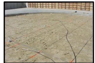
MMO Ribbon Anode Grid CP System
