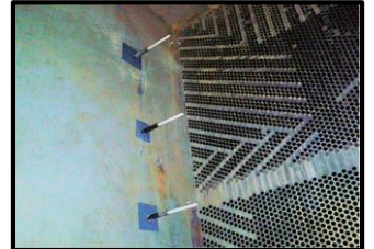
ICCP Anode in Condenser Box
