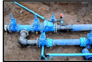
Fire hydrant Piping
