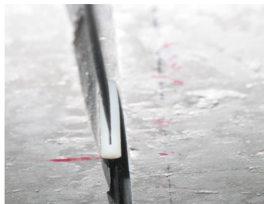
Ribbon mesh in saw-cut slot
