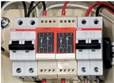
Heavy-duty lightning surge protection modules for AC& DC and AC&DC breakers
