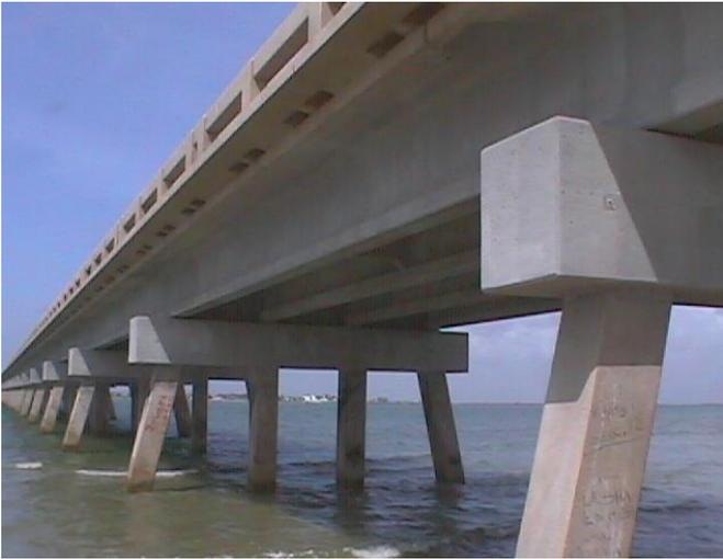
Figure 8. Thermally sprayed Al-Zn-In anode for galvanic cathodic protection of a concrete bridge.
