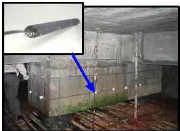
Figure 4. Titanium discrete tubular mesh anode installed in the pile cap in Hong Kong.
