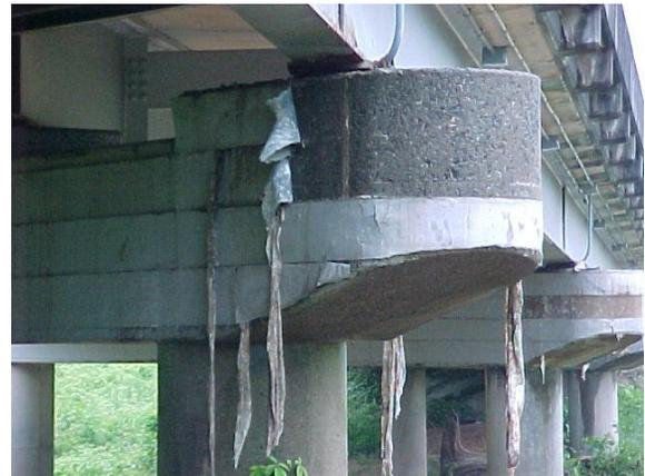
Figure 4. Zinc anode failure
