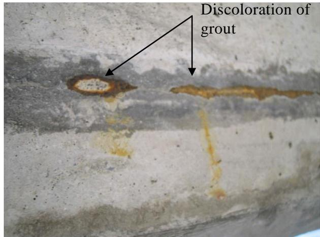
Figure 6. Discoloration of the grout by the reaction
