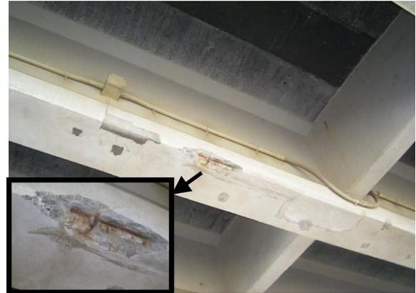
Figure 2. Concrete spalls after the discrete anode CP system was installed.
